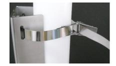
2. Wind Stainless Belt around the pole, pass the belt end through the metal fittings, and wind up Stainless Belt by the adequate torque.
