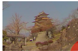
Partial enlargement (80m ahead) Monitoring with high resolution all the way around far
